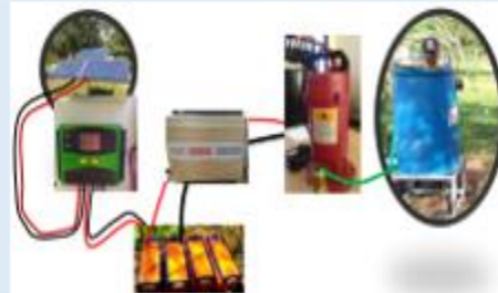
Picture 3: AC pump installation
